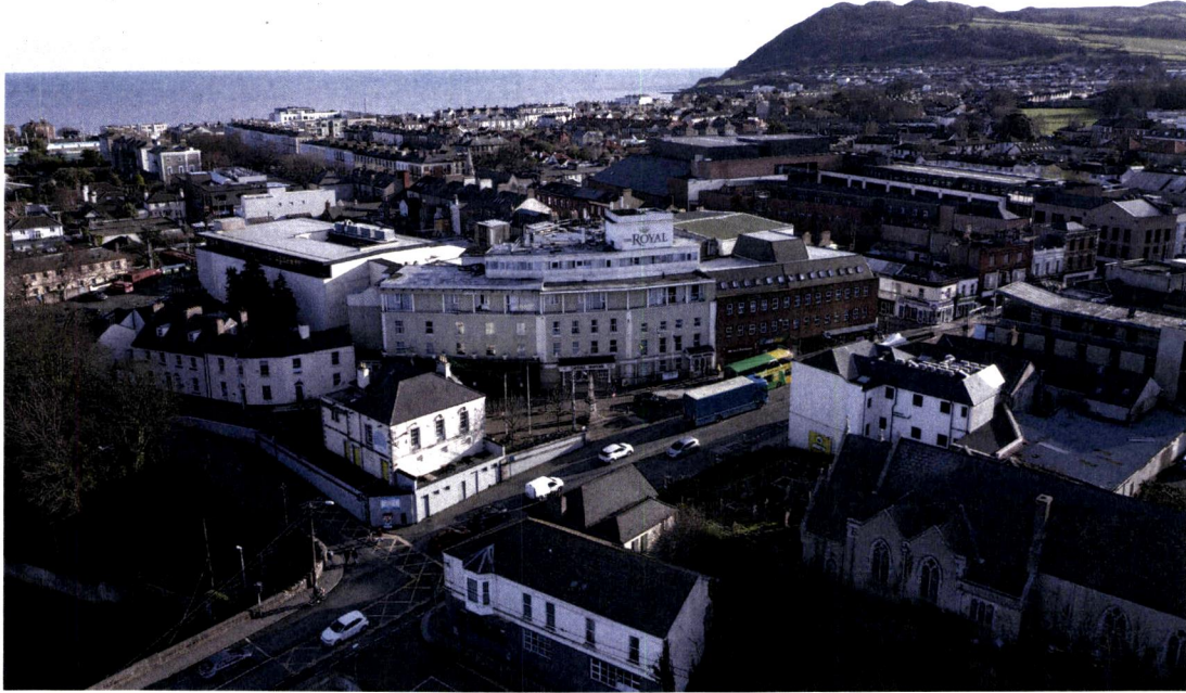
Photograph A – View from West
